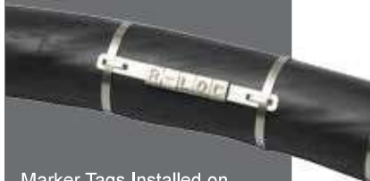
Marker Tags Installed on Power Cable
